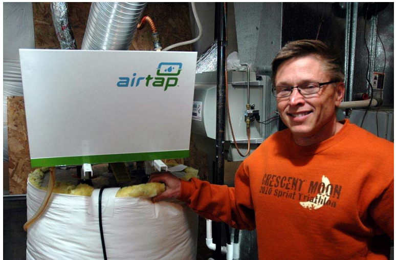
Greg shows us the AirTap heat pump water heater. It uses ambient air in the AirTap and stores the heated water in a standard electric water heater below the AirTap unit.
