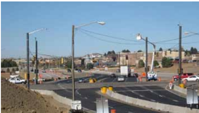
The current configuration on Parker Road at Arapahoe Road looking north.
