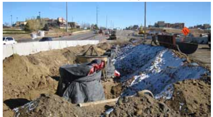
Crews have started constructing the pier columns for the new Parker Road bridge over Arapahoe Road.
